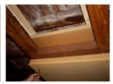
9. Now, install GUTEX Thermosafe-wd with tongue and groove edge profile over the Multiplex-top prior to installing the air barrier/ vapour barrier.
