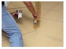
4. Apply GUTEX Voranstrich primer to the GUTEX sarking board and allow to flash off.
