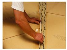
6.Affix GUTEX adhesive tape to the GUTEX sarking board, being careful to avoid air blisters or wrinkles. Press through the tape to flatten the caulking.
