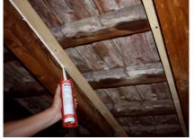
7. Fill the joints between batten and rafters with GUTEX caulking along the entire length of the joints.
