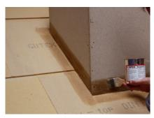
I.Apply GUTEX Voranstrich primer to the GUTEX sarking board and adjacent material surfaces and allow to flash off.
