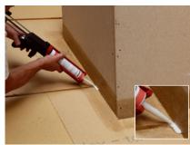
2. Fill the joint with sufficient caulking material.
