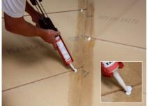
5. Fill the joint with a sufficiently large bead of GUTEX caulking.
