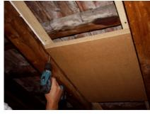
8. Fasten the GUTEX Multiplex-top boards to the batten. Make sure the boards are pressed tightly to the batten.
